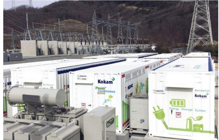
Kokam 56 MW Energy Storage at South Korean
